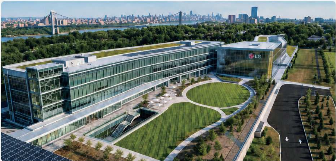
LG Electronics North America Headquarters in New Jersey
