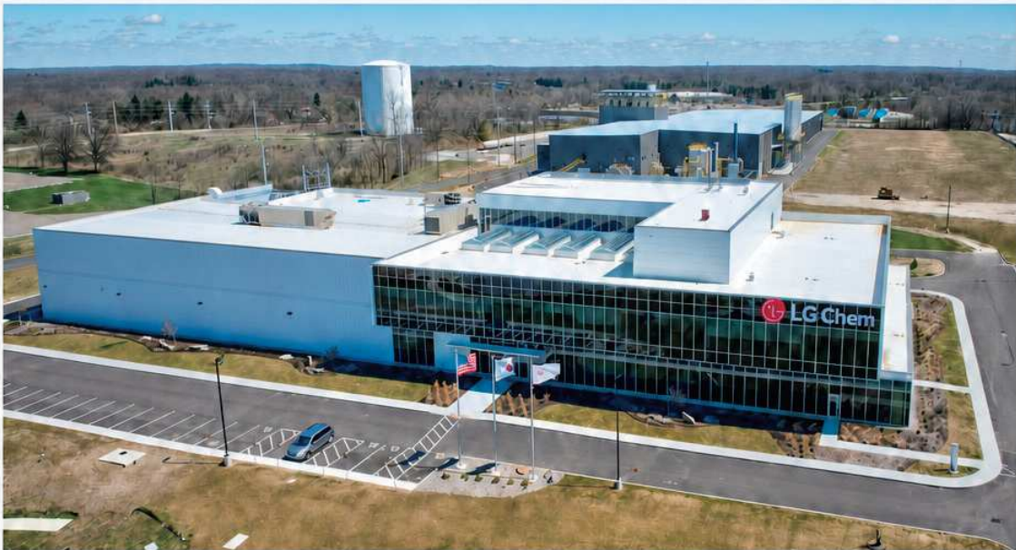
LG Chem Customer Solution Center in Ohio
