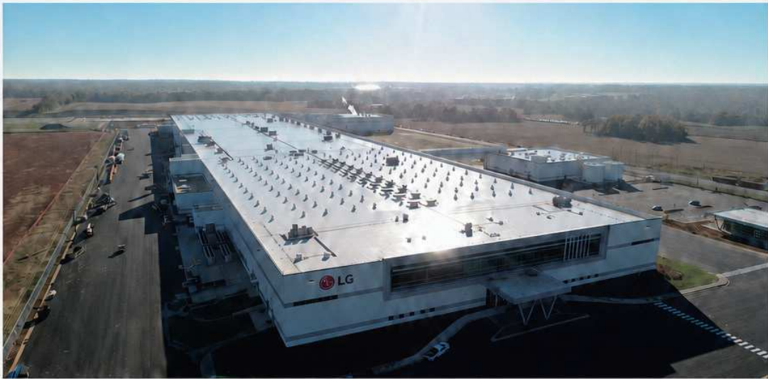
LG Electronics smart laundry factory in Tennessee
