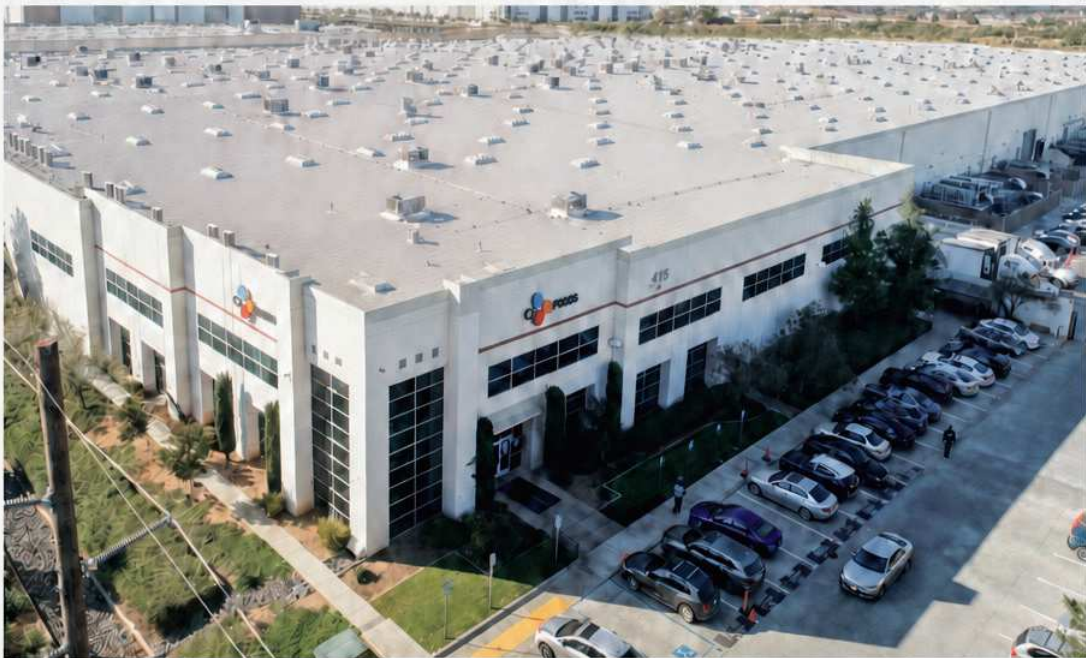
CJ CheilJedang's production facility in California
