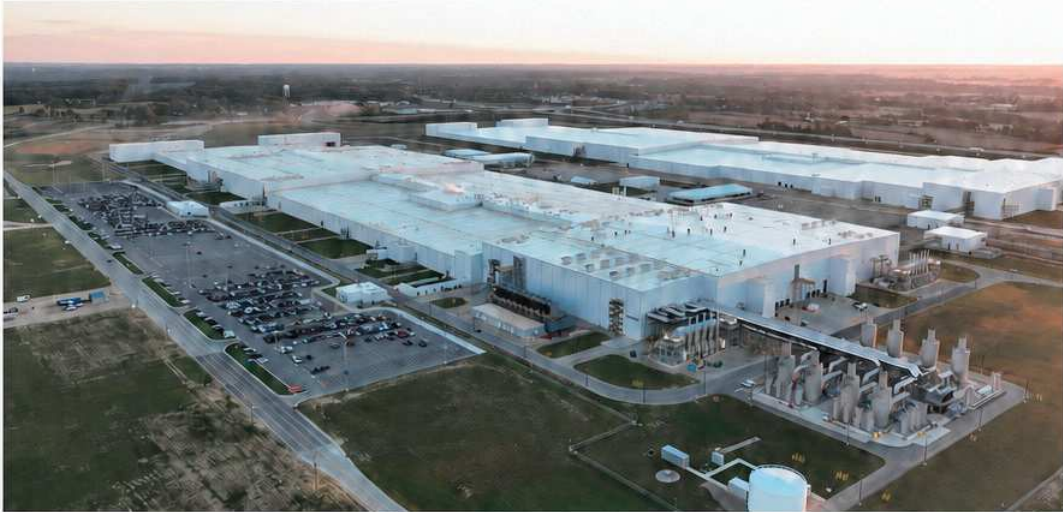
BlueOval SK Battery Park in Kentucky
