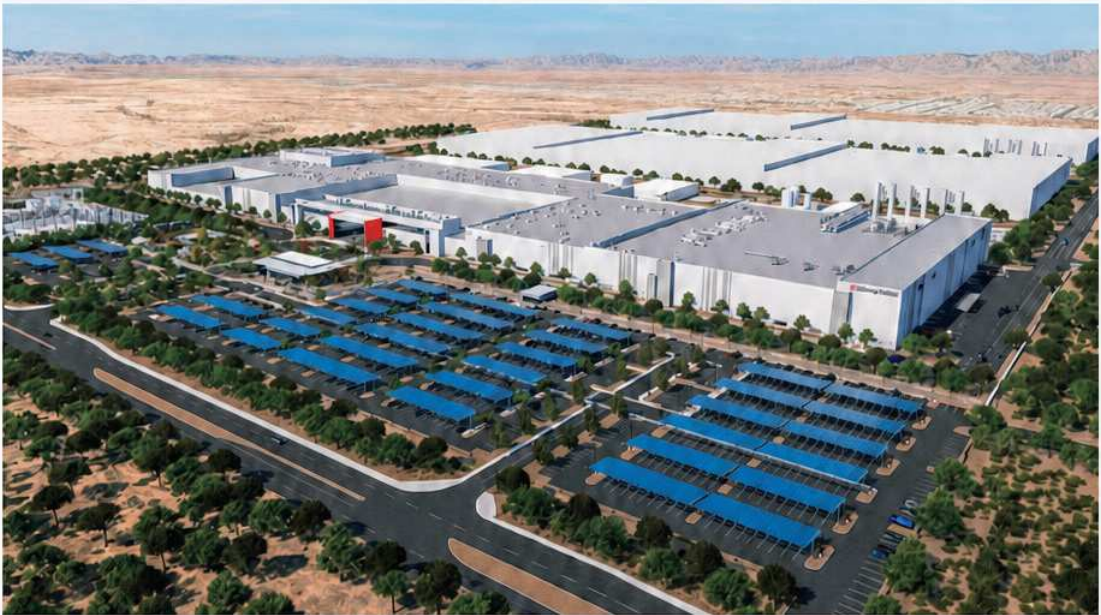
LG Energy Solution's battery plant under construction in Arizona
