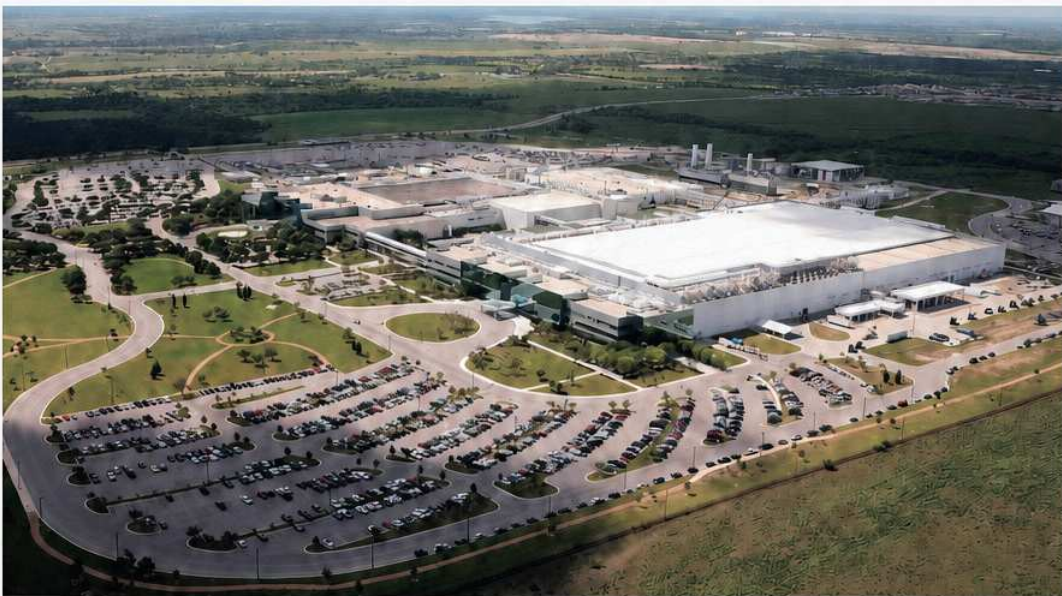
Samsung Electronics semiconductor manufacturing plant in Texas
